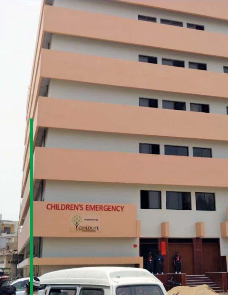
ChildLife's Children Emergency Room, Abbasi Shaheed Hospital.
